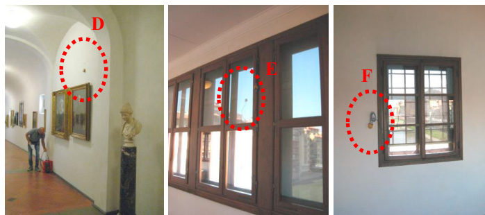
Figure 2. Photographs of the data loggers in positions D, E and F.
