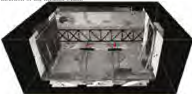
Three-dimensional images of the point cloud with identification of the insertion of the metallic beam.
