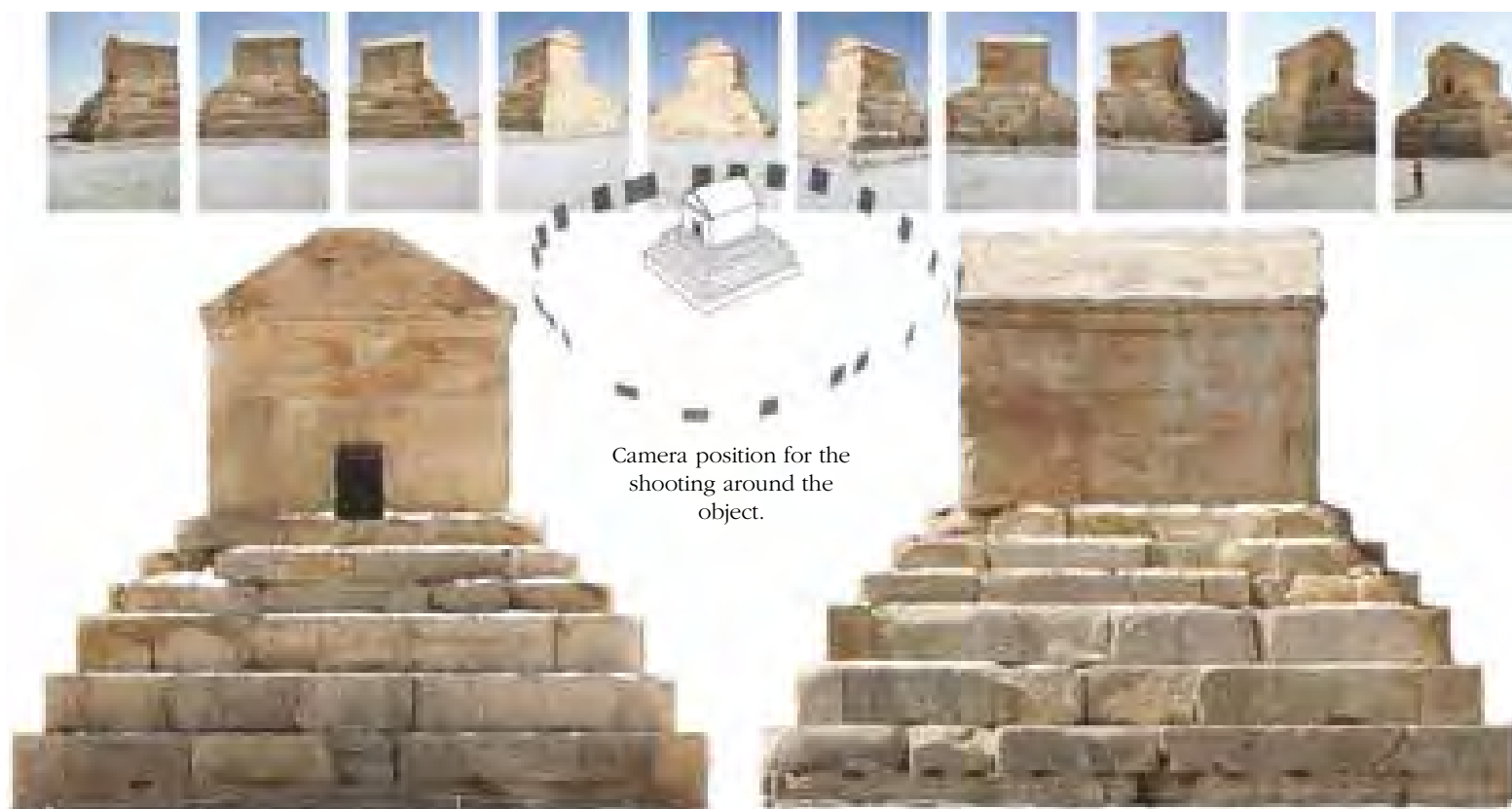
Elaboration of two-dimensional faces of the Tomb of Cyrus the Great. The model, suitably scaled on three points of the basement measured on site, has allowed to realize a photographic three-dimensional elaborate highly reliable and responsive to reality.
