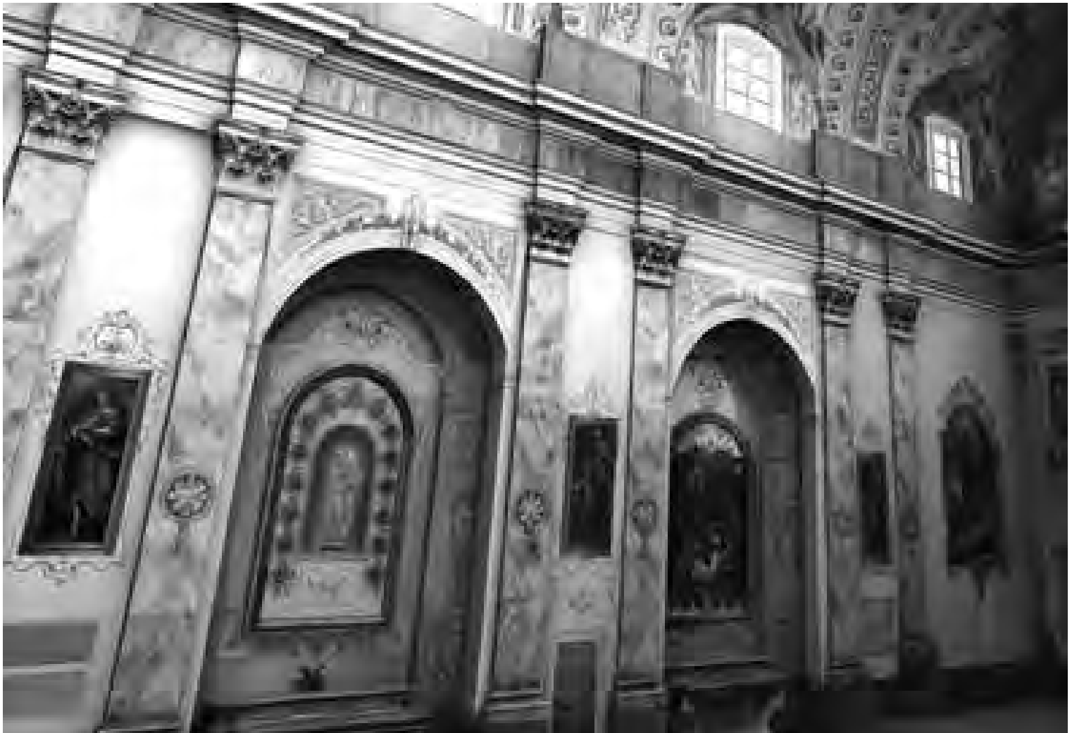
Views of 3D models: virtual urban landscapes (opposite page), and the inside of the Church of the Monastery of Camaldoli (Above). The spatial complexity of the volumes and the quality of the materials make the models the effects of hyper reality.
