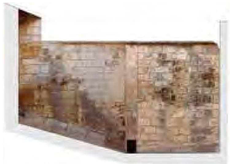
2d vectorial drawing and photo mosaic of the North Corner, north side. In this case the state of conservation can be evaluated. On the left side shows a whole area of loss stones, filling with concrete material.
