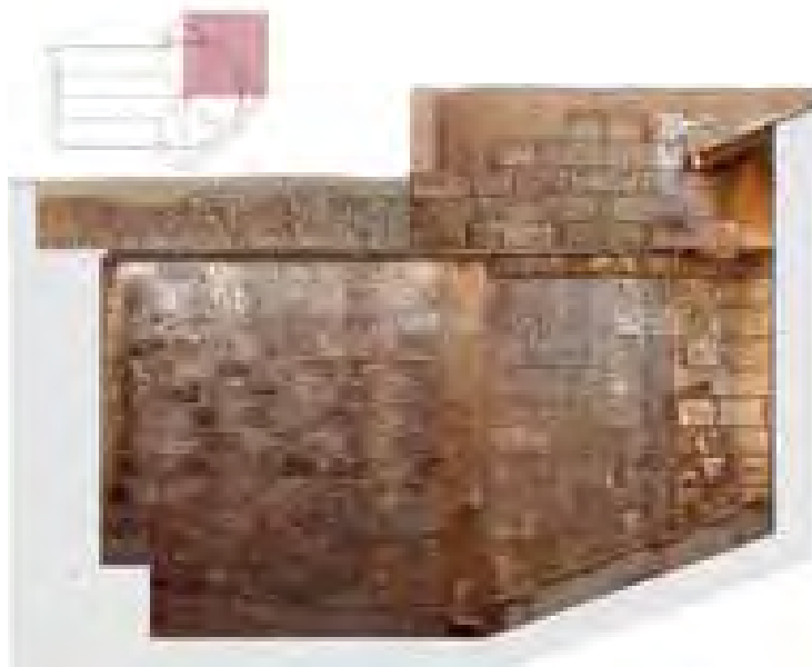
2d vectorial drawing and photo mosaic of the North Corner, east side. As per the upper pictures, in this case the state of conservation can be evaluated. The chromatic alteration is due to the microbiological attack and to the rain-water action.
