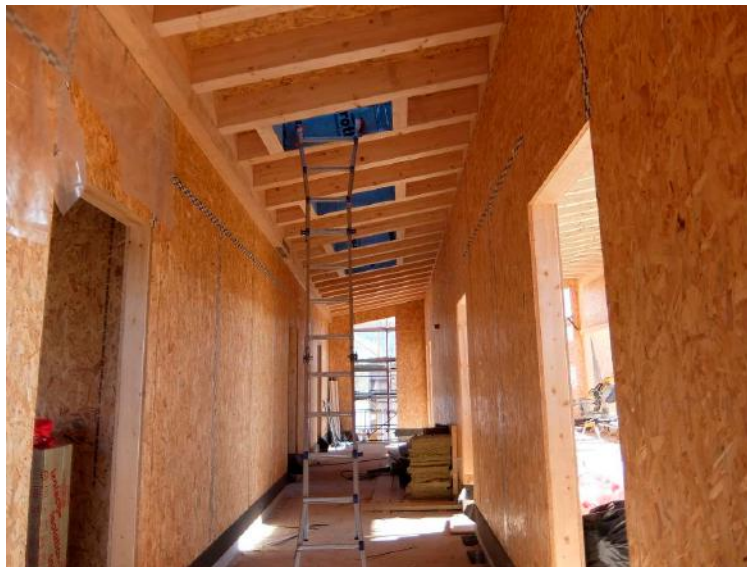
Figure 5. Hallway of the building under construction.
