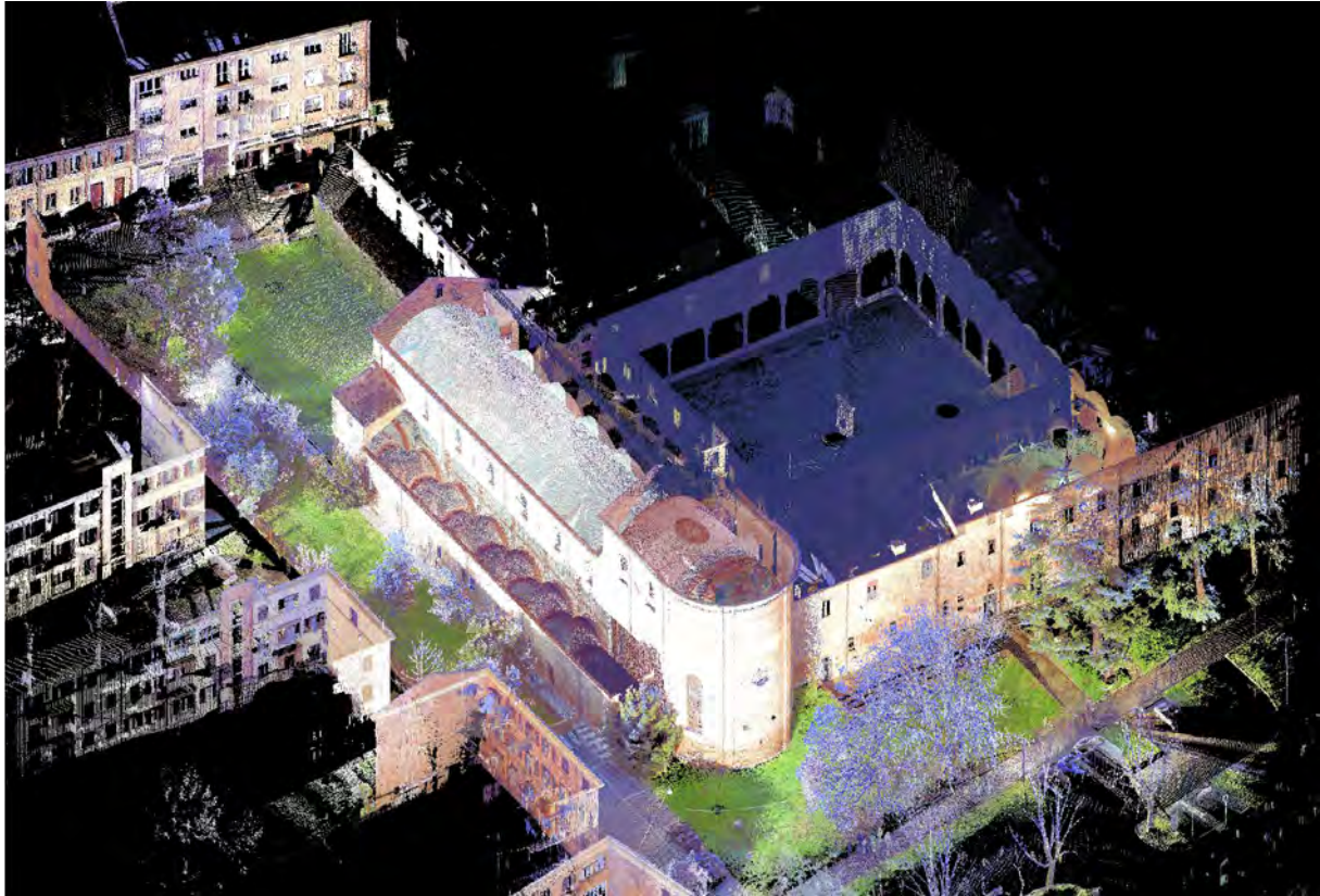
Fig. 1 : The church of Santa Maria della Consolazione in Ferrara. isometric view of the point cloud model obtained by matching 52 scans in Faro Scene and then importing the whole model in Cyclone.
