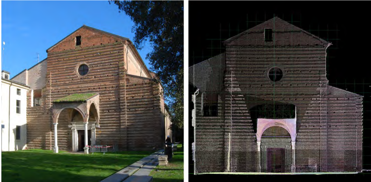
Fig. 2: Front of the church of Santa Maria della Consolazione in Ferrara. From left: photos during survey campaign and screenshots extracted from PointCloud.
