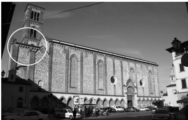
Figure 1. San Domenico church (Prato, Italy): localization of the vaulted room.
