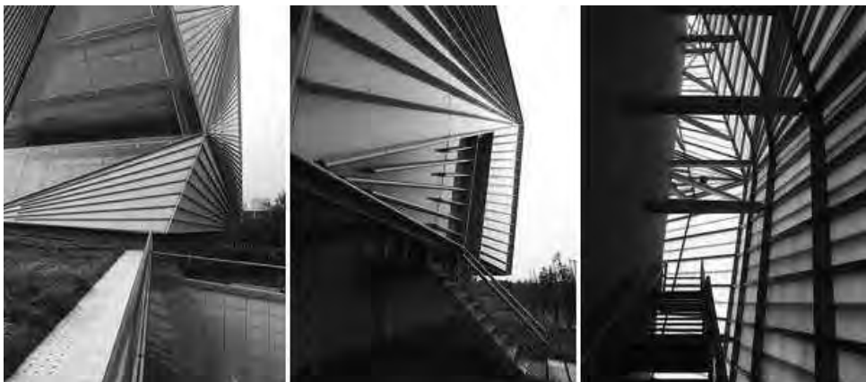
Fig. 1.3: CSET, Centre for Sustainable Energy Technologies, Mario Cucinella Architects, Ningbo, China, 2009
