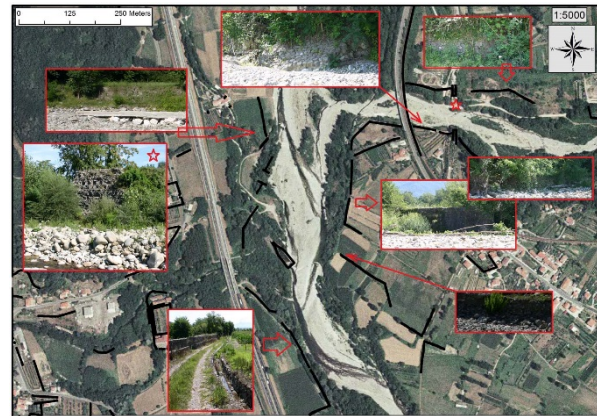
Fig. 2 Some nineteenth-century agrarian settlements have resisted better than the latest engineering works to the flood of 2011 (Magra River Basin in Tuscany).
