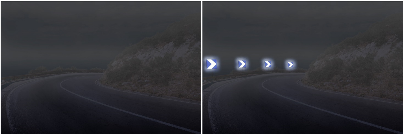
Fig.6 Pictures show the different visibility in the same place between hairpin during the night with fog and during the night with fog but with LSCs panels integration.
