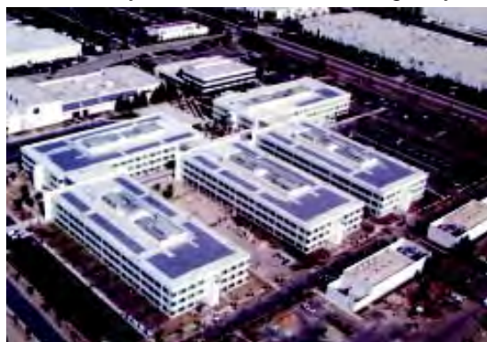
Fabbrica Toyota in California, Powerlight System
