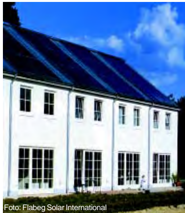
Foto: Flabeg Solar International
