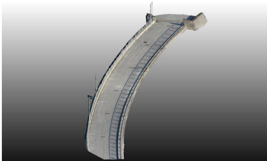
Figure 2.2. Texturized 3D mesh of the road way on the dam crest.
