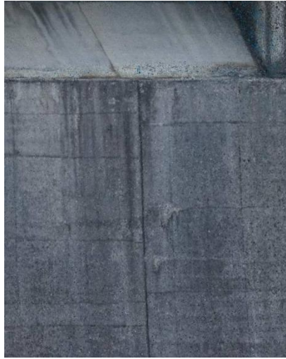
Figure 2.11. UAV Dense Point Cloud. A small variation such as joints can be recognized by the RGB information associated with the points.
