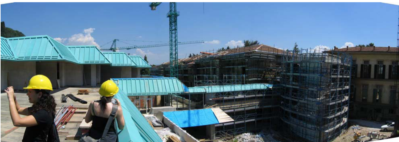
Fig. 1 A technical vist to a construction site
