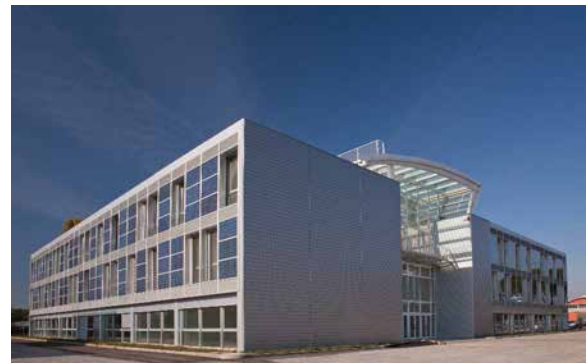
► Fig. 1: The Domino facade was used in the construction of the south and east façades of the New Centre in virtual environments and ICT of Lucca Chamber of Commerce.
