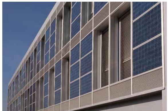
► Fig. 2: The south façade of the ICT in Lucca. In this case, three PV panels generating an electrical energy production of 0.30 kWp are integrated into the opaque module of the DOMINO façade.
