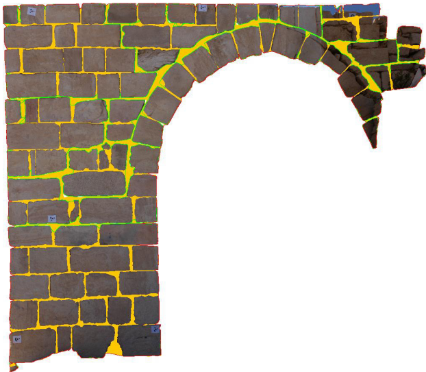
Figure 12. Orthophoto generation on a query related to blocs, with design of USM perimeter and the cement paint in yellow.
