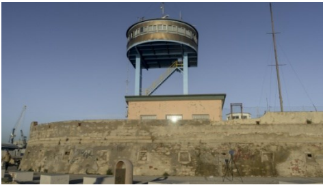
Fig. 2- The “capponiera” with the tower of maritime control service (Anna Frascari, 2018)
