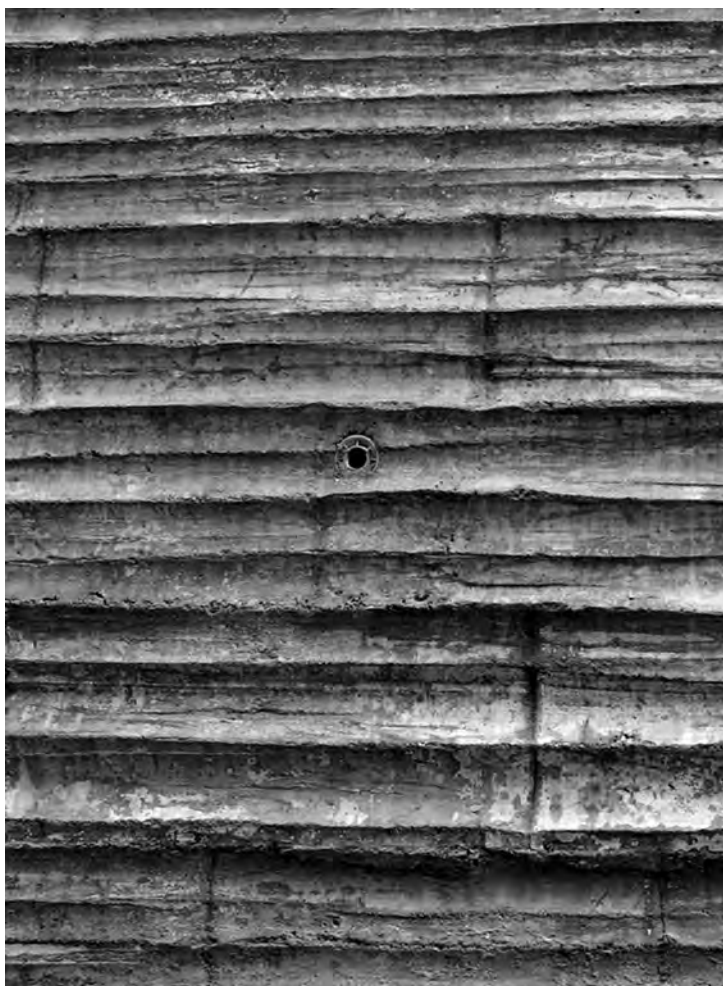
Amateur Architecture Studio, Ningbo Historic Museum , Ningbo (Cina) 2008, parete c.a. (photo: Yding Yang).
