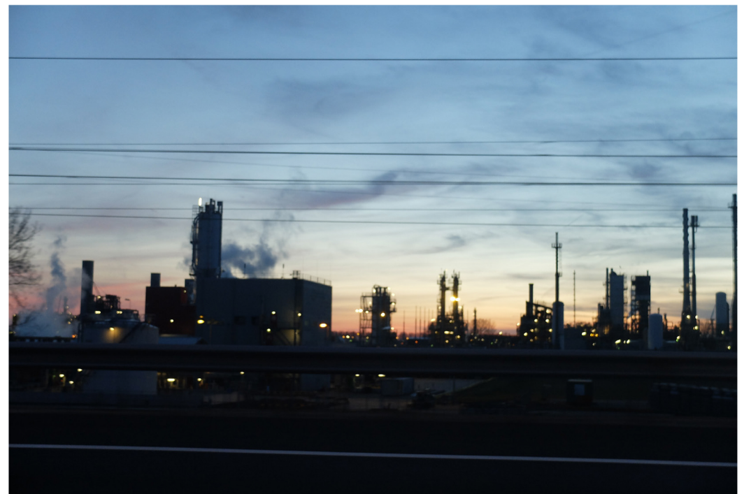
Fig.2 - View of the port of Rotterdam where the structures and productive activities of the port prove to be incompatible with the city
