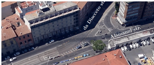
Figure 8.2: Aerial view of the Diacceto-Alamanni intersection.
