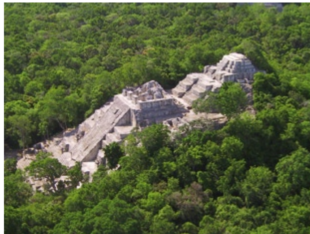
Fig. 2 Aerial view of Structure II.
