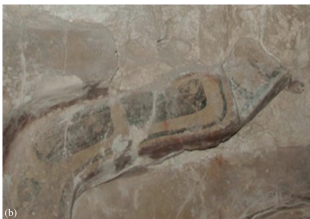
Fig. 4 Polychrome-modelled stucco in sub-structure II C-1 of the Gran Plaza: (a) before restoration; (b) post-restoration. Re-adhesion of detached fragments was performed using an autogenously air-setting mortar.
