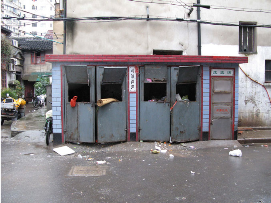
Fig. 7.5 Installation for the pre-sorting of household waste in a Shanghai district. Photo S. Barles, January 2008
