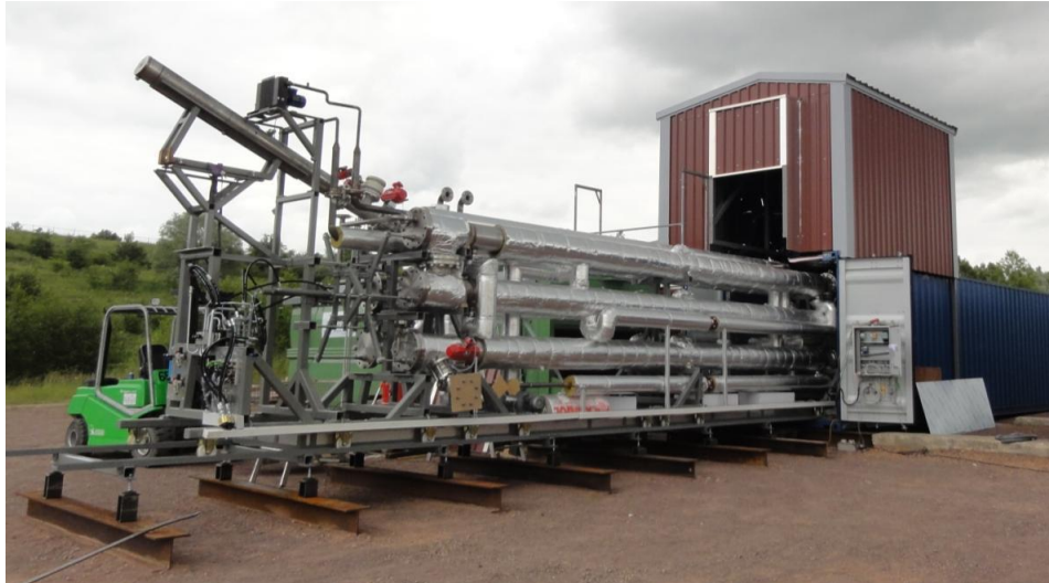
Figure 23: Artcoal 3000k plant in Halle, Germany [94].
