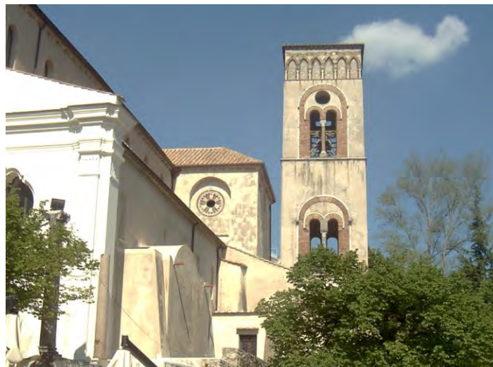
Fig. 7: Ravello, Cathedral, Bell tower
