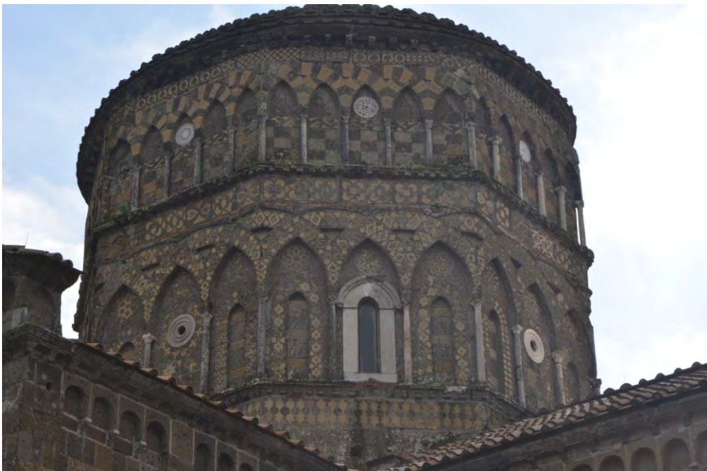
Fig. 14: Casertavecchia, Cathedral, Lantern tower
