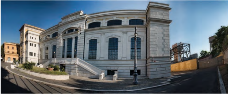
Figure 1 - The façade of the Montemartini power plant develops the main front inside the lot in an open area. On the top central part there are the carved characters SPQR ( Senatus PopulusQue Romanus , “The Roman Senate and People”), which connects the new building to the tradition of the public work from the Roman Age.
