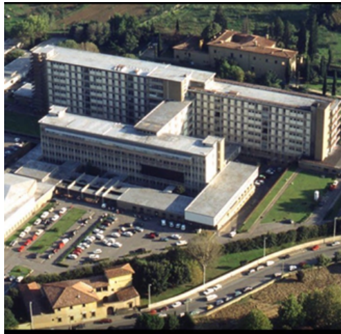
Figure 6.20: Picture of building
