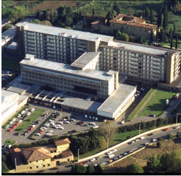
Figure 5.17: Picture of building
