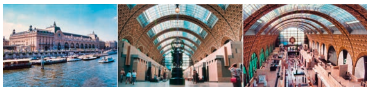
Figure 10 - The Gare D'Orsay in Paris: view of the front along the Seine; views of the interior; main pavilion.
