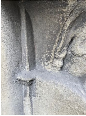
Figure 1.9 Black crust (sheltered area)
