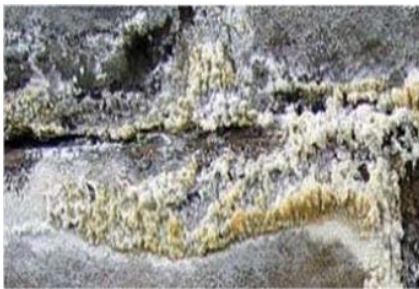
Figure 1.11 Efflorescence
