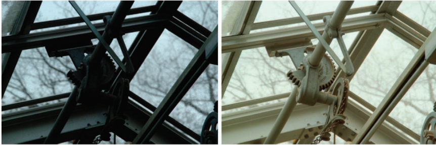
Figure 2.4: Example of SDR (left) and HDR (right) captures taken while camera was facing light source and capturing an object against it [4].
