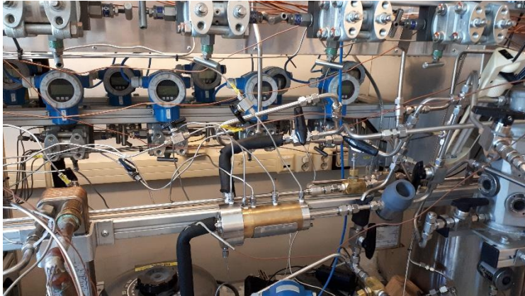
Figure 94 Ejector assembled and mounted in the test-rig
