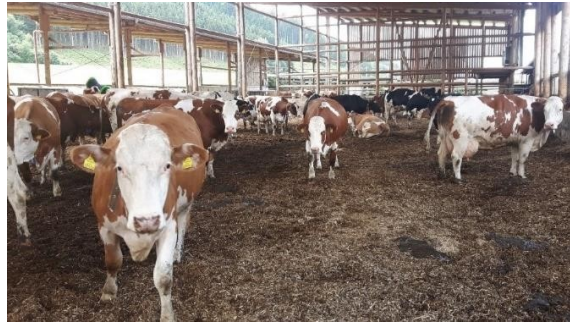
Figure 5. An Austrian compost barn with timber structure.
