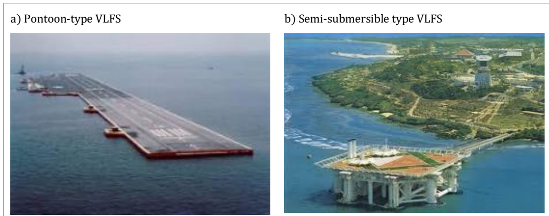
Fig. 2.2 - a) Pontoon-type VLFS (the floating airport Mega Float in Tokyo Bay, Japan) and b) Semi-submersible type VLFS (the floating city Aquapolis in Okinawa, Japan)
