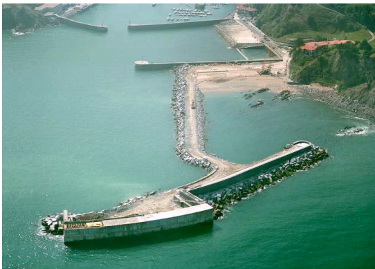
Mutriku plant 16 OWCs 296kW, Spain
