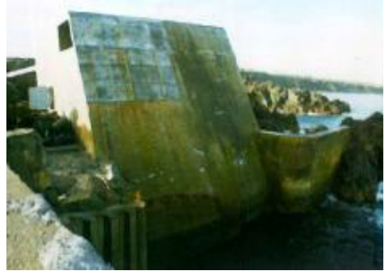
Pico Plant - 400kW Portugal.
