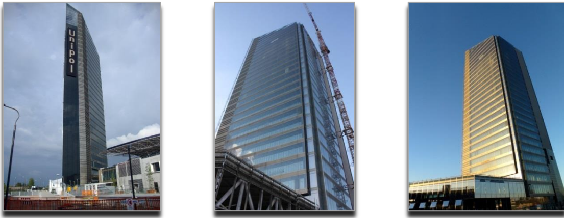
Fig. 1.6 - A case study with characteristics of the selected reference façade typology: the Unipol Tower in Bologna (Italy). Pictures of the tower under construction (left, center) and completed (right).
