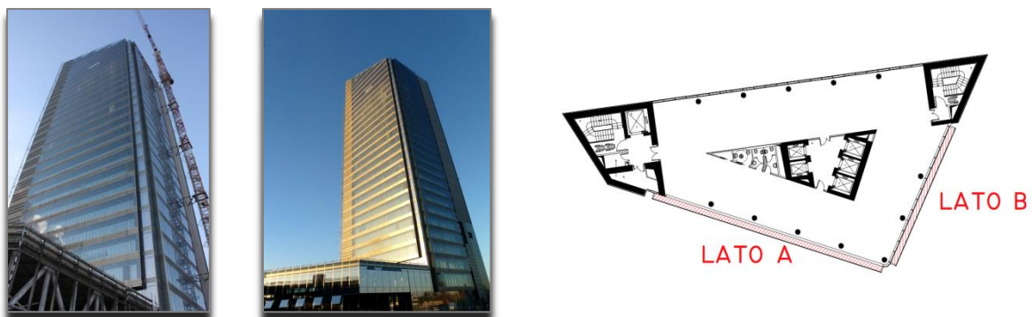
Fig. A1.35 - Practical example of building envelope with horizontal compartmentation: the Unipol Tower (Bologna, Italy). In this case the building is equipped with a permeable envelope on two building sides. View of the two double-skin façades during the construction (left), and at the end of construction (center). On the right, a horizontal section with the two façades is highlighted. Courtesy of Permasteelisa Group.
