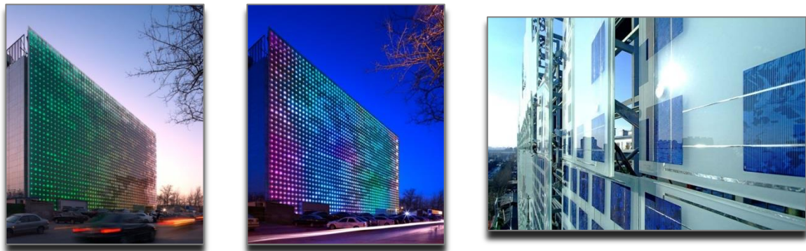
Fig. A1.39 - An application of building envelope with porous screen: the GreenPix zero-energy media wall designed by Simone Giostra and partners (Beijing, China). Font: www.archdaily.com .
