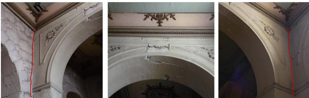
Figure 5.2.8—In-plane behavior of the transverse arcades
