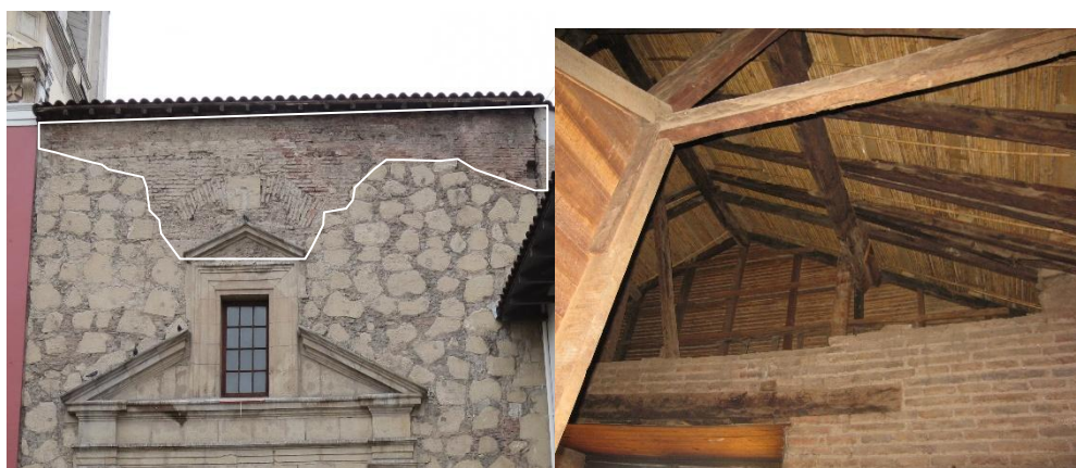
Figure 5.2.10 –Upper part of façade and presbytery wall.
