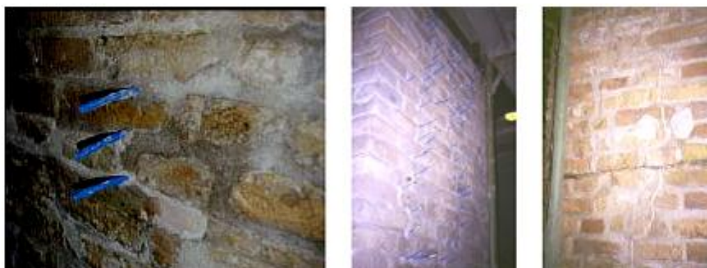
Figure 6.14 – Grout injections (Source POLIMI-UNIPD)
