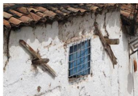
Figure 6.1 - (a) Tie beams in the Kuño Tambo church, one of the prototype buildings of the SRP (image by C. Cancino, 2010); (b) exterior view of connections of tie beams in Cuzco (image by S. Lardinois, 2012).
