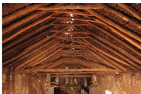
Figure 6.1 - (a) Tie beams in the Kuño Tambo church, one of the prototype buildings of the SRP (image by C. Cancino, 2010); (b) exterior view of connections of tie beams in Cuzco (image by S. Lardinois, 2012).
