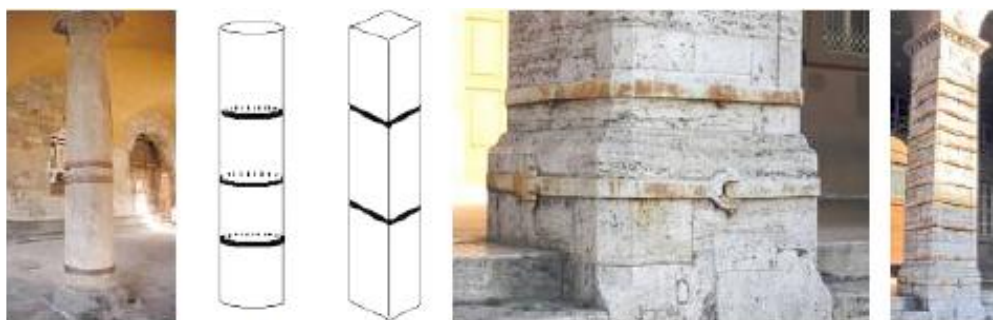
Figure 6.18 – Confinement of column and pillar (Source UNIPD)
