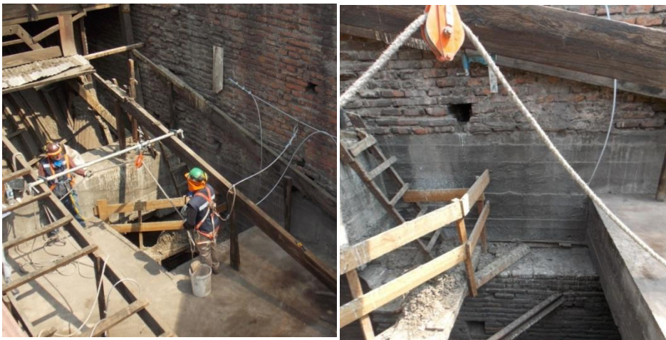
Figure 5.3.12 - RC slab located above the arches of the narthex
