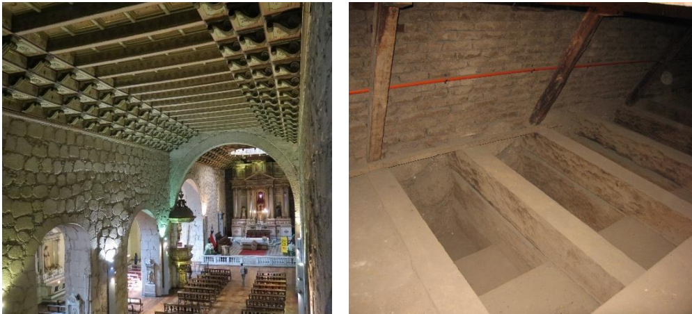
Figure 5.2.7 - Horizontal diaphragm placed on the central nave
