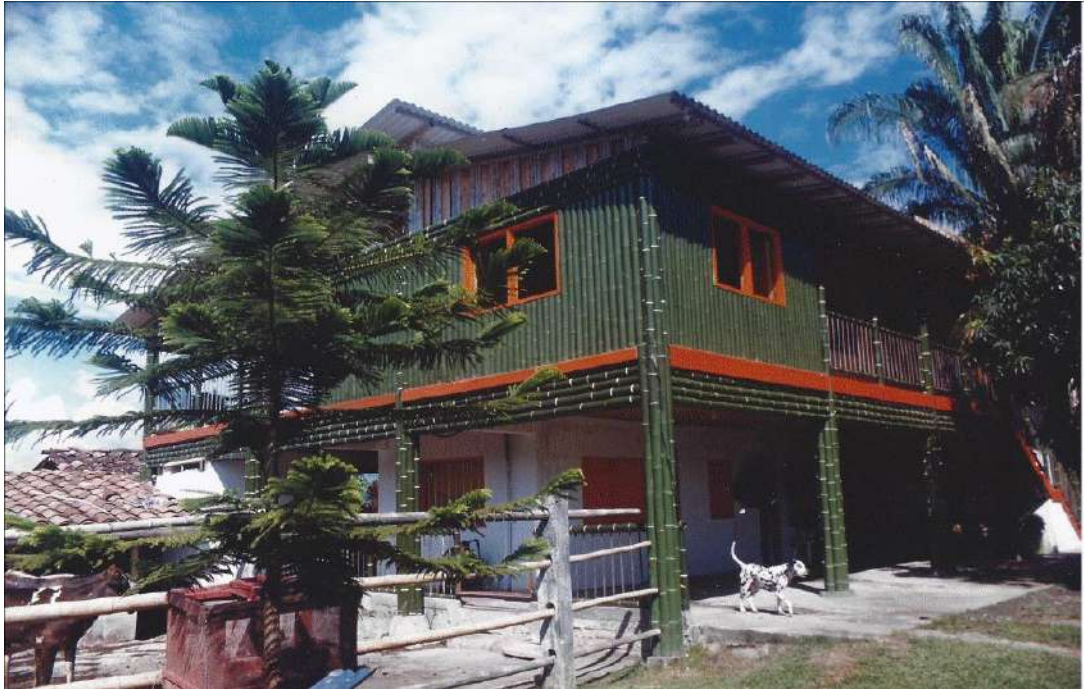
Fig. 1 Case of study, house reinforced with bamboo in the Colombian coffee region
