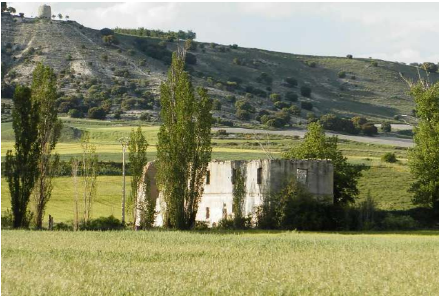
Fig. 2 Pineapple of Esgueva. Valladolid. Spain. Old hydraulic mill
