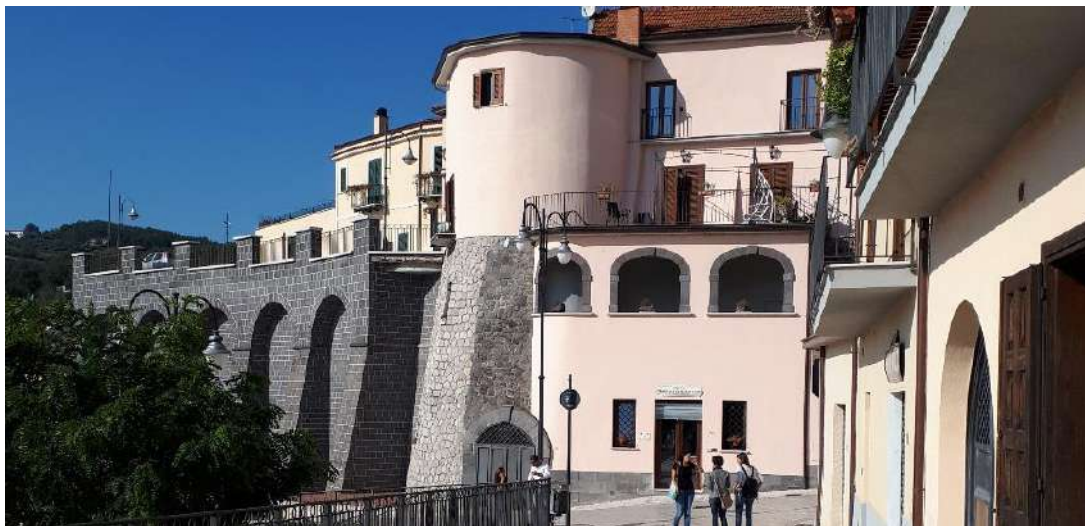
Fig. 1 View of Ruviano small town (CE) Italy
