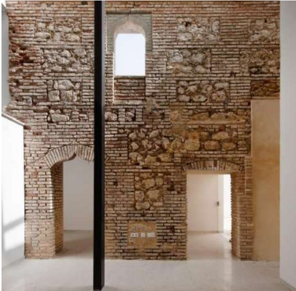
Fig. 1 García Torrente Arquitectos. Refurbishment of three old Mudejar houses into 18 social housing. Carmona. Sevilla
