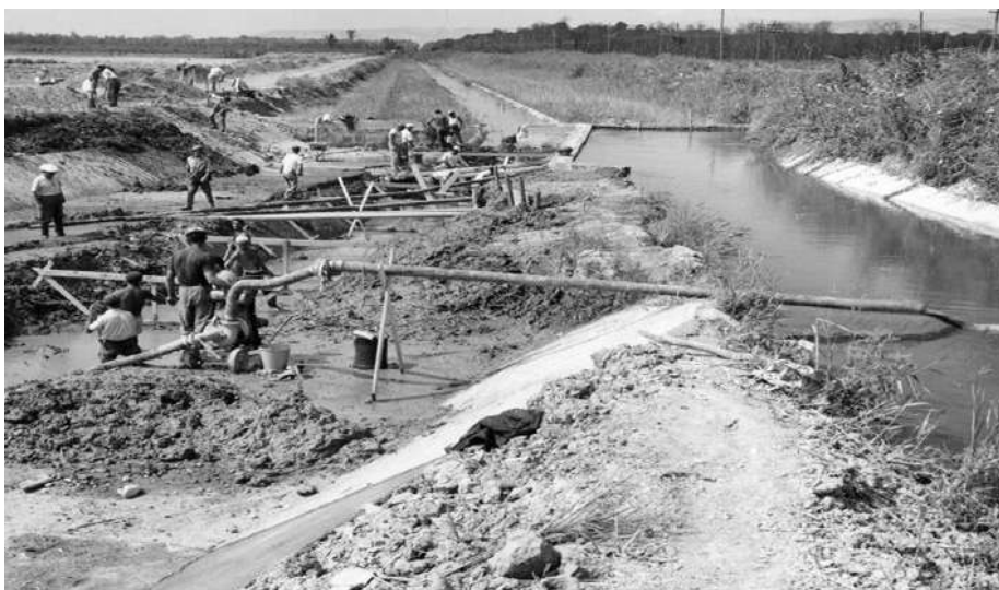
Fig. 2 Historical image of reclamation processes in “Borgio Pianelle”
