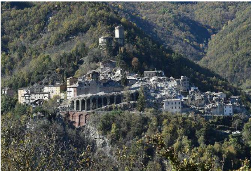
Fig. 2 Arquata del Tronto, province of Ascoli Piceno. The village after the 2016 earthquake
