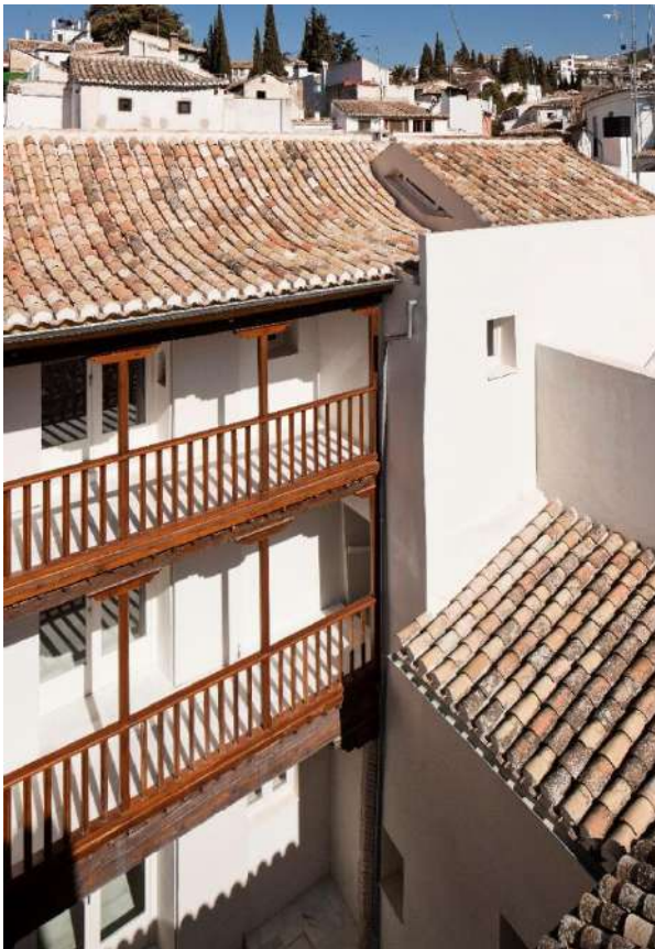
Fig. 2 García Torrente Arquitectos. Refurbishment of Casa Zayas into 8 social housing. Albaicín, Granada
