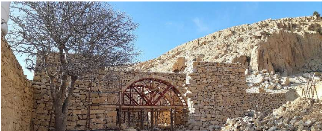
Fig. 2 Part of the rehabilitation works at al Matan Village
