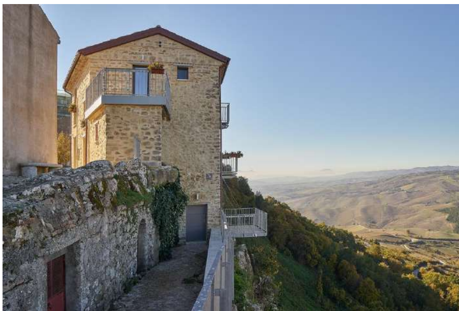
Fig. 2 Cairano, house on the cliff, northern facade
