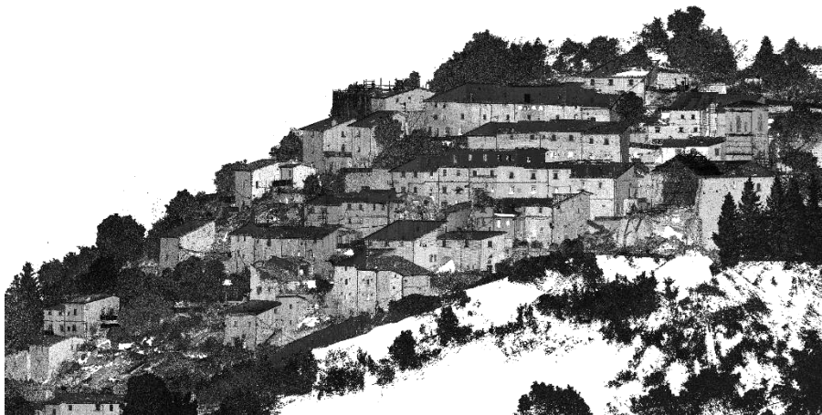
Fig. 2 Campi di Norcia (PG) a panoramic view of historic centre
