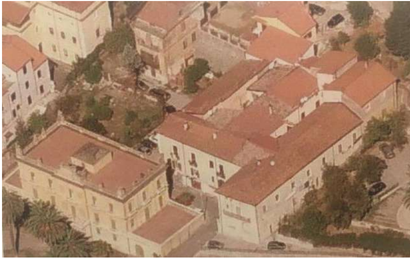
Fig. 1 Colle Triglio, province of Cosenza: a panoramic view of the Villa Rendano and the Textile Mill
