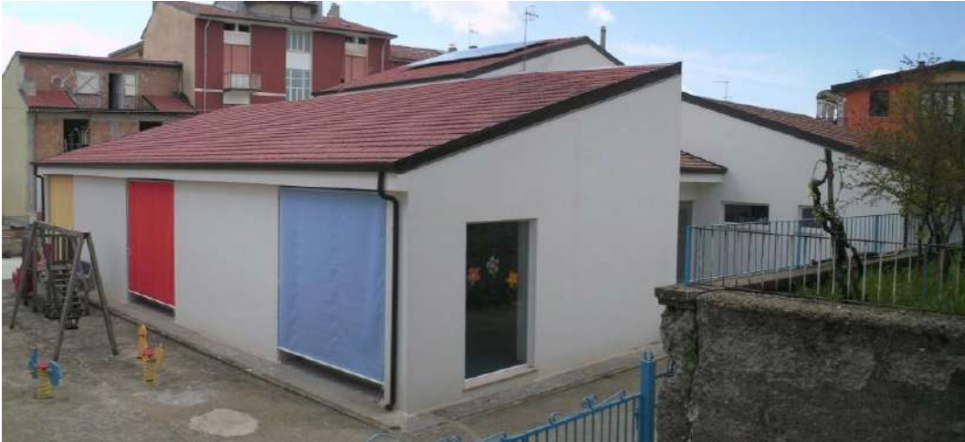
Fig. 1 Perspective of the building with classroom in the foreground
