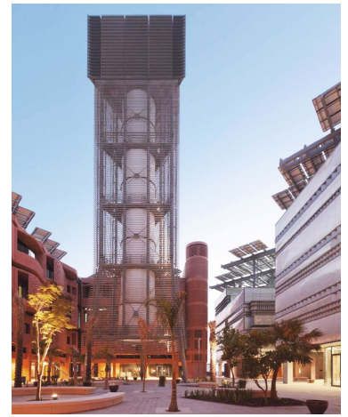
Foster & Partners, Torre del vento , Masdar Institute, 2010.
