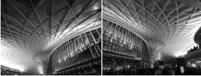
Figure 4. The Large Shelter Designed Using Parametric Software in the King's Cross Station Main Hall (pictures by Elliott Brown).
