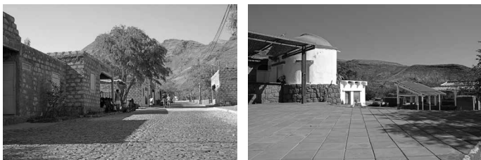
Fig. 4-5. Lajedos, a remote community in the island of Santo Antão. Cape Verde. Communal workshop for blocks production; photovoltaics panels that generate electricity for several buildings of the community (photos: M. Pereira and Â. Lopes — Atelier Mar).
