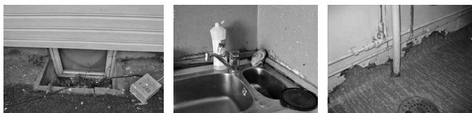
Fig. 2. Examples of low standard and moisture problems in decentralized reception centres. Left: Sleeping room window with insufficient daylight conditions (photo: K. Denizou). Middle and right: Worn down surfaces and moisture in kitchen and bathroom (photos: R.Ø. Thorshaug).
