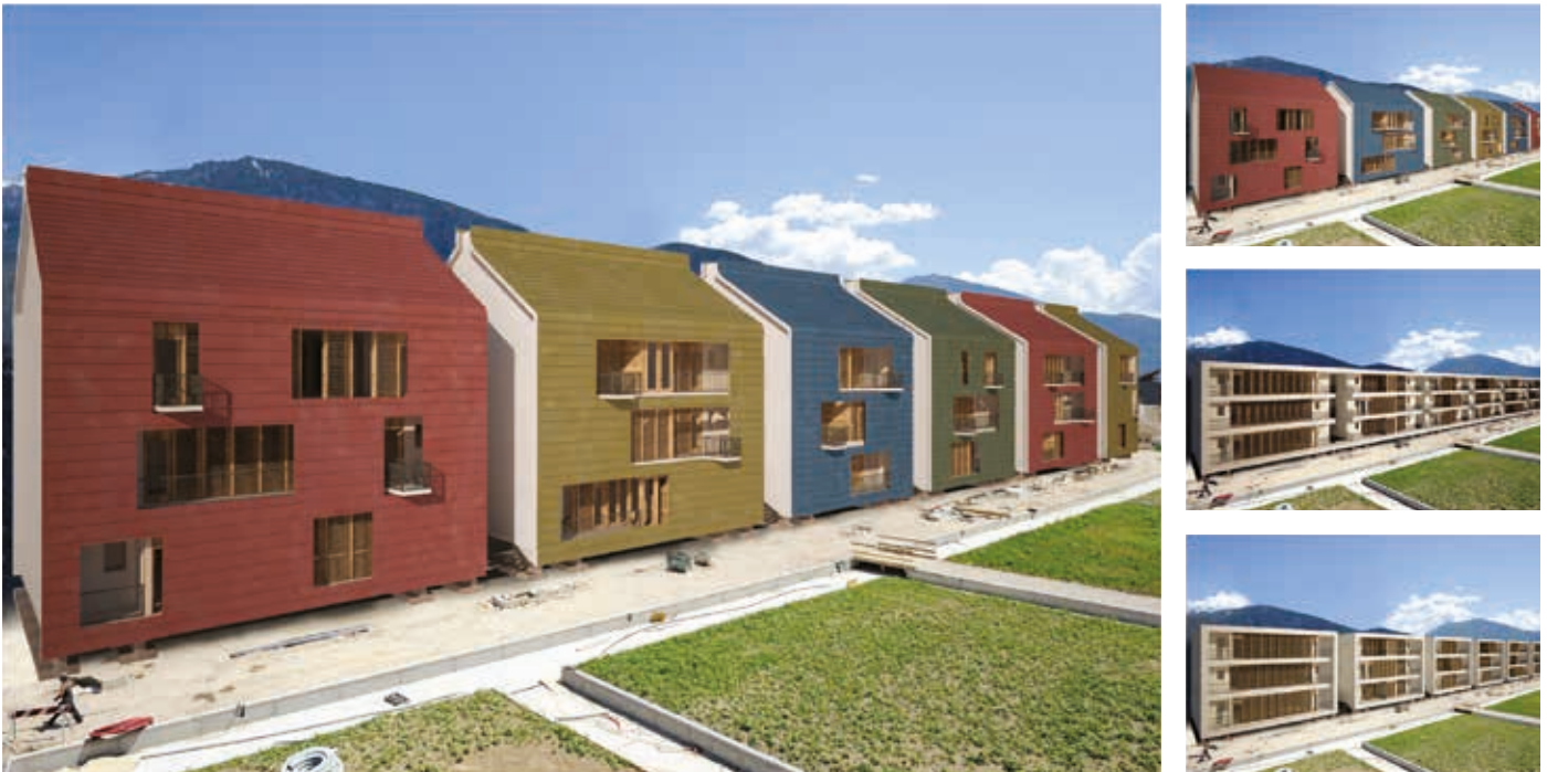
Figure 8. Possible external views of the S.A.T.O.R. Project, depending on the shell definition.
