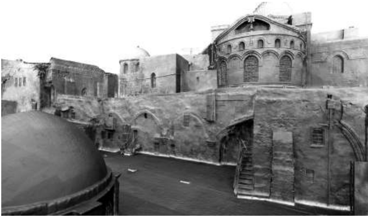
FIGURE 2 3D mesh model: view of the Apse of the Katholicon from the area above the Chapel of St. Helena, (L. Fiorini, from point cloud surveyed by Tucci-Bonora).
