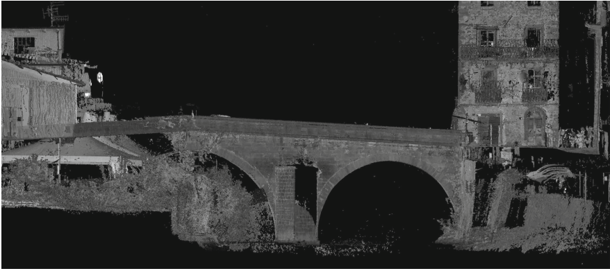
Fig. 6. The image represents the digital survey by laser scanner of a medieval bridge in Garfagnana, a mountain locality in the province of Lucca in Tuscany.
