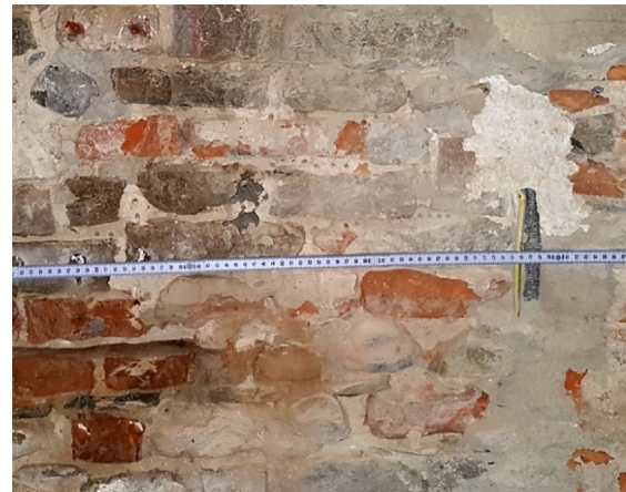
Fig. 15. Case study n.3. Window of masonry after plaster removal.
