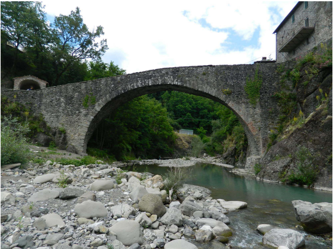
Fig.6 View of the San Michele Bridge
