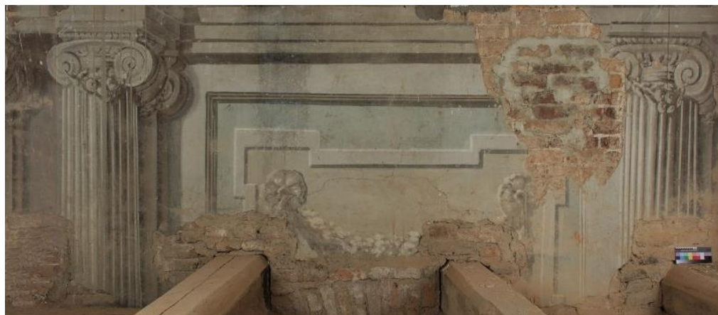
Figure 2. The area upon which the pilaster sided entablature was leaned
