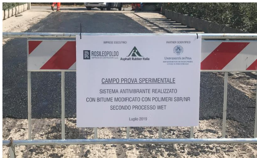
Figure 6.18 Construction bulletin board
