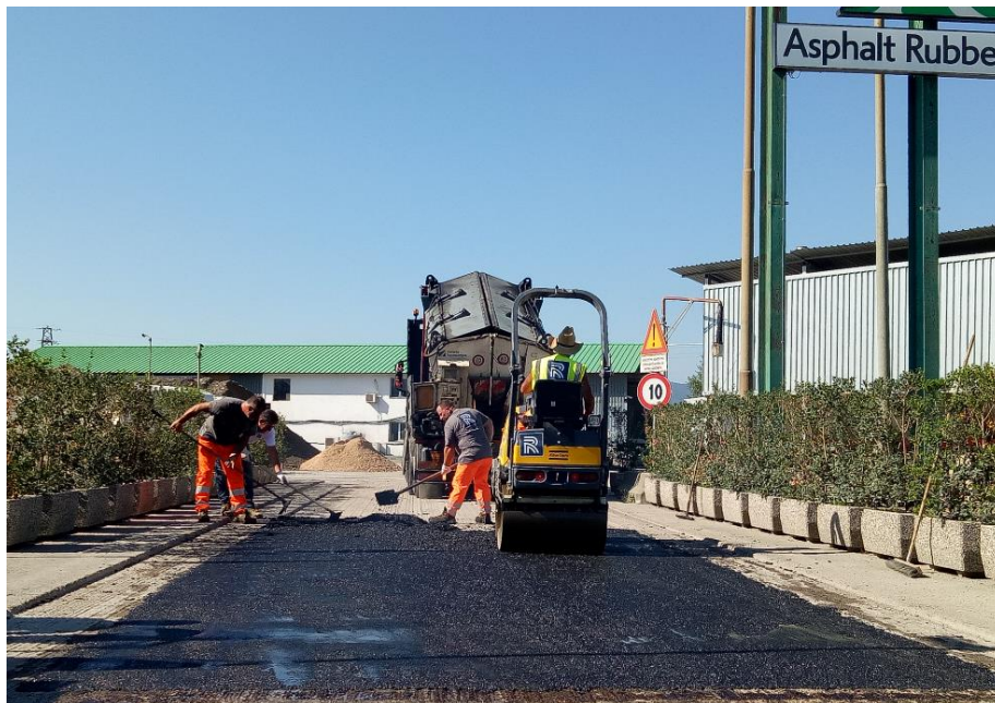
Figure 6.21 Paving process of the damping layer
