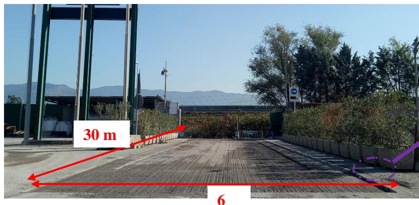
Figure 6.19 The old asphalt pavement
