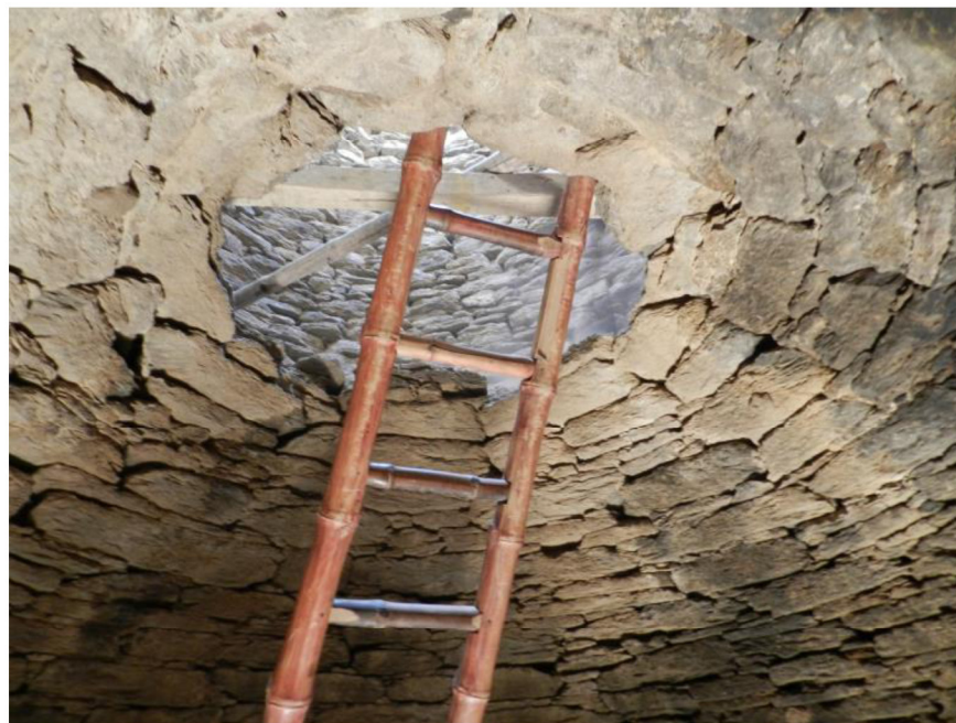
Figs. 3-4 - Conservation in progress (below: a detail of the double domes). (Photos by F. Martore).
