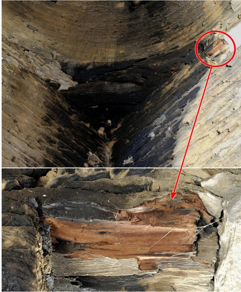
Figs. 10-11- Particular of the sampling point from beam 4, on the SE corner. (Photos by E. Loliva, processed by GG).
