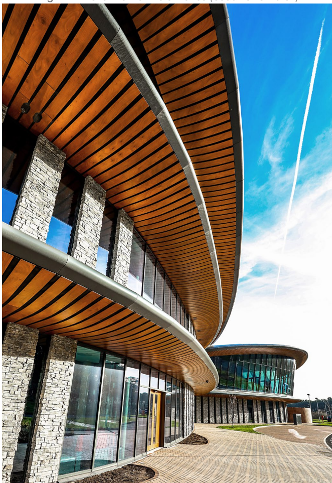
Fig 42 Exterior view of the entrance (Caudwell Children)
