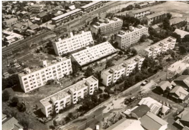
Figure 2.1: Tilted buildings as a consequence of liquefaction after Niigata Earthquake (from website: depts.washington.edu ).
