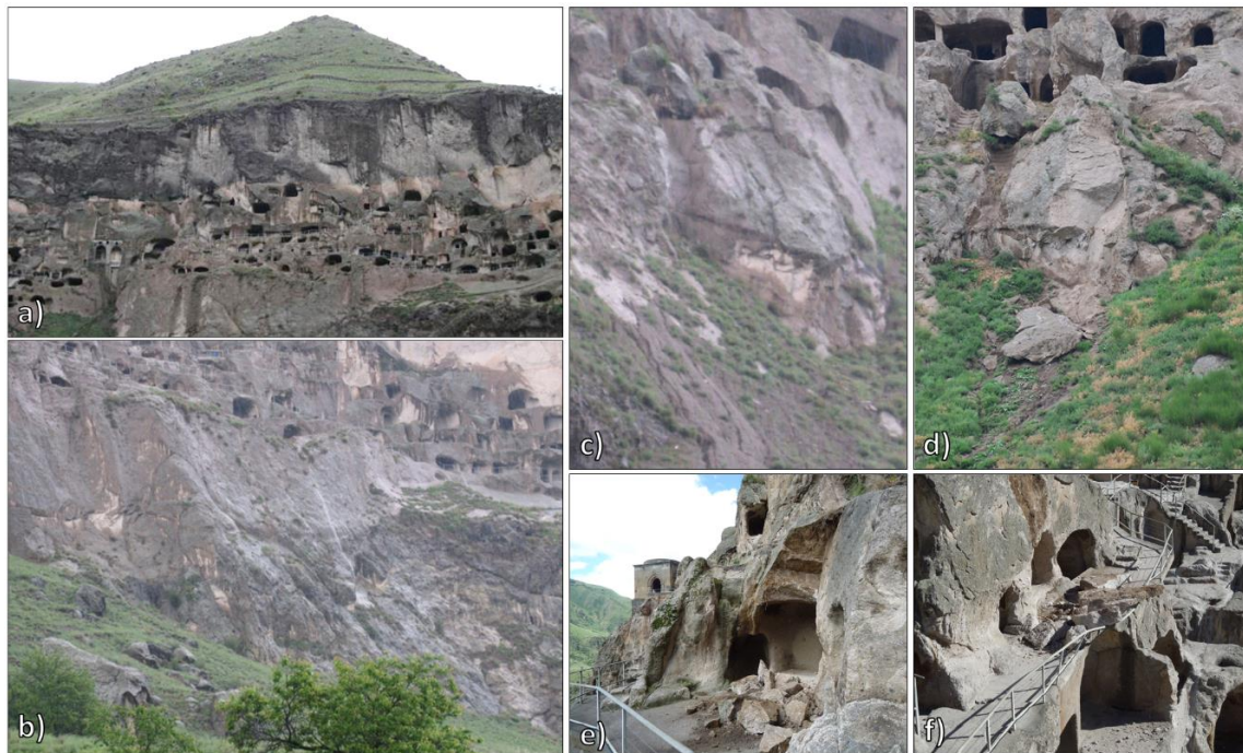
Figure 14. Conservation criticalities due to water runoff-infiltration: intense water runoff during a rainfall event in 23 May 2014 on the slope face (a) and slope toe (b) (courtesy of the director of the site), detail of collapsed block in AOI5 (c: before the collapse – photo taken on 25 May 2015) and after the collapse (d). Details of rock collapses occurred after rainfall events: 11 July 2016 (e) and 19 September 2016 (f).
