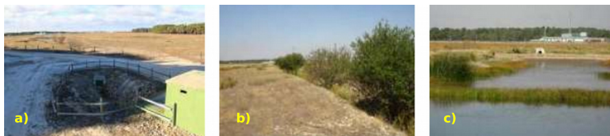
Figure 8.4: "Triplet" components: (a) infiltration pond; (b) bio-filter in a MAR channel; (c) artificial wetland.
