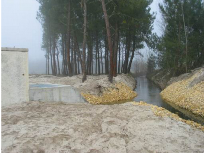
Figure 8.6: Arroyo Ternillo with recharge water.
