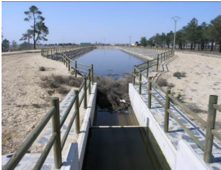
Figure 8.7: Infiltration lagoon near Gomezserracin.
