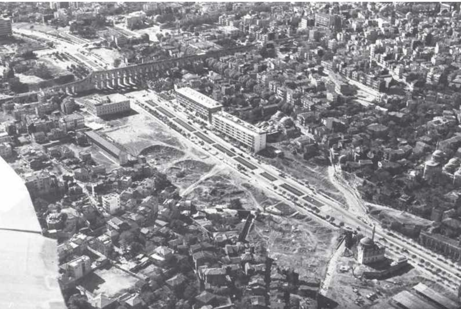
The Atatürk Boulevard with the ancient Valente's aqueduct
