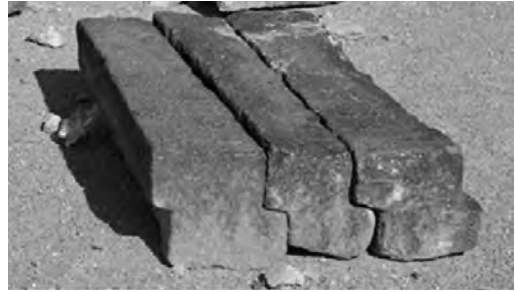
Fig. 18 – Single-chaired voussoirs from Qasr Al-Hallabat (Jordan), Umayyad architecture, VII AD ca. (Giuliani, 2011).
