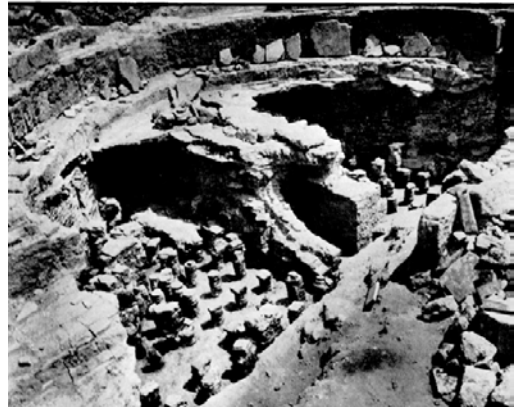
Fig. 8 – The hypocaust of the semi-circular pool in Salamis central caldarium before the restorations (Karageorgis 1968).
