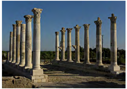
Fig. 4 – Restored southern end of the Colonnaded Street of Soli Pompeiopolis, in the area where the street was connected to the port. Image courtesy of Mezitli Municipality.
